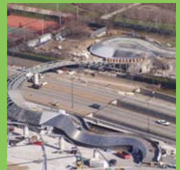
Imperial Construction Associates erected the sections over Columbus Drive in one weekend. Cladding was done by Permasteelisa and Radius Track.
