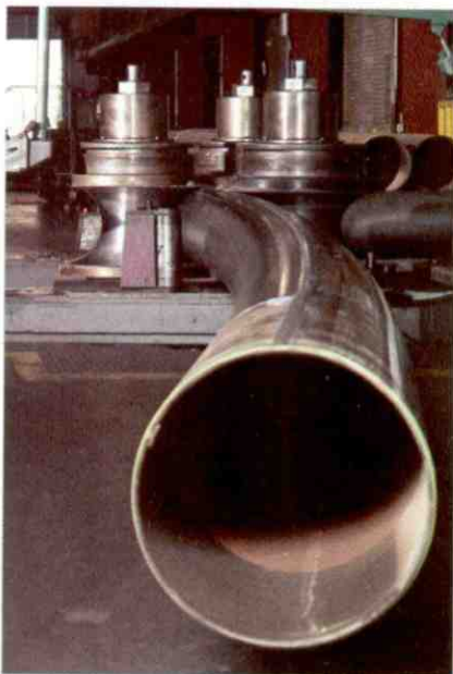
The arena curtain-wall's 16-in HSS steel is curved in the fabrication shop. 2009 IDEAS 2 Awards: Chicago Metal Rolled Products
