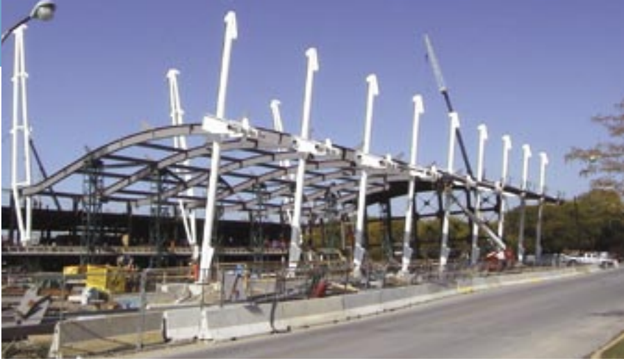
Photos for this article courtesy Chicago Metal Rolled Products.
