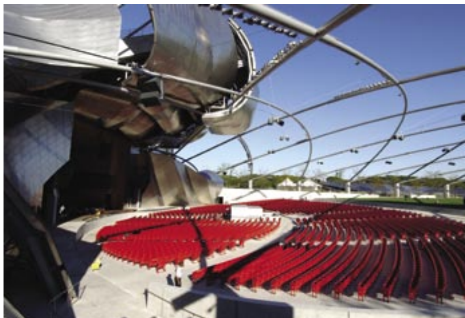
The trellis geometry for the Jay Pritzker Pavilion in Chicago was slightly modified to simplify fabrication and erection and to reduce costs.
