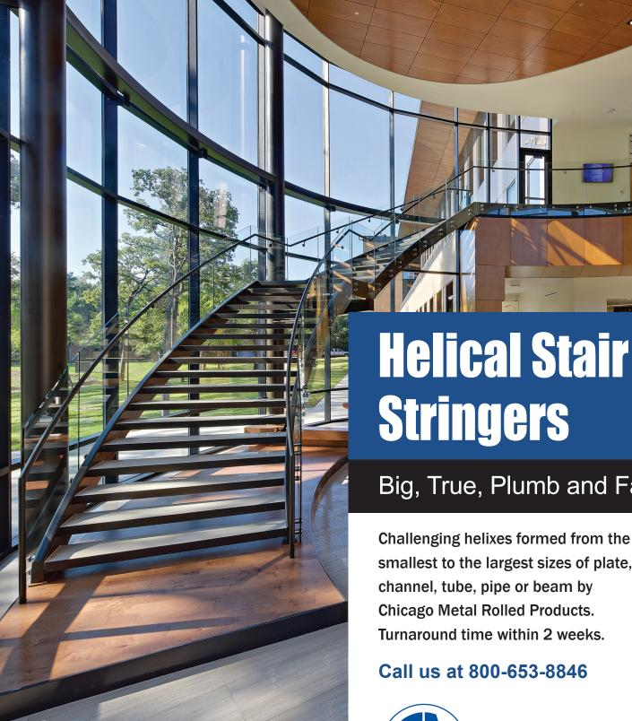
12 x 3 x 5/16" rectangular tubes curved the easy way to a 12' inside radius (inside stringer) and an 18' 1" inside radius (outside stringer).
