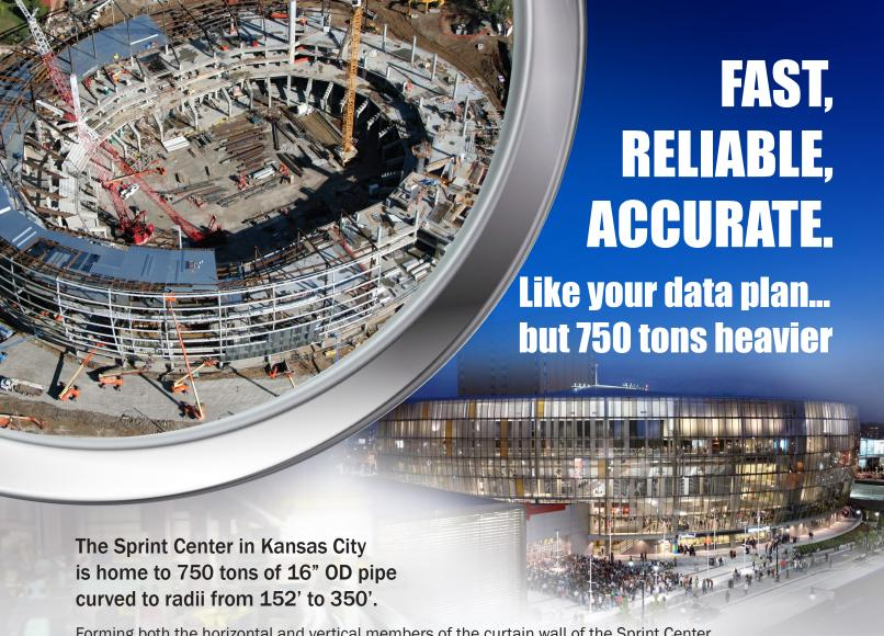
Forming both the horizontal and vertical members of the curtain wall of the Sprint Center, the curved steel frame is *held to tolerances tighter than those of the AISC Code of Standard Practice*.
