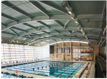
Chicago Metal created **16 reverse curves** of W33x169# beams, cold bent on the x-x axis, each without a \$1,500 weld splice. A total of 310 tons of curved beams form the wavy roof of the Ratner Athletic Center at the University of Chicago, winner of the AISC Engineering Award of Excellence.
