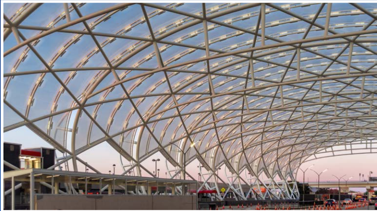
2020 IDEAS 2 National Winner - 920 pipe members rolled from 1300 tons of 14" pipe creating 38 super-trusses for the iconic canopy at Hartsfield-Jackson Atlanta Intl Airport. Atlanta, GA
