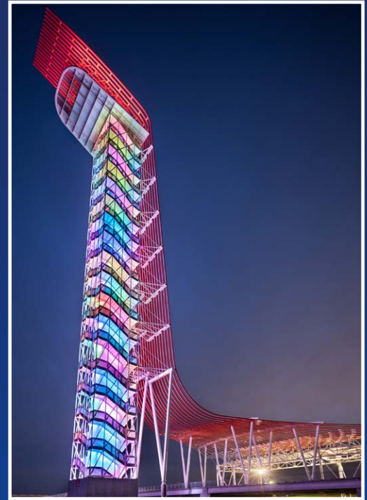
2015 IDEAS 2 Merit Award - 73 pieces of curved 8" sch 40 pipe totaling 35 tons for Circuit of the Americas Observation Tower. Austin, TX
