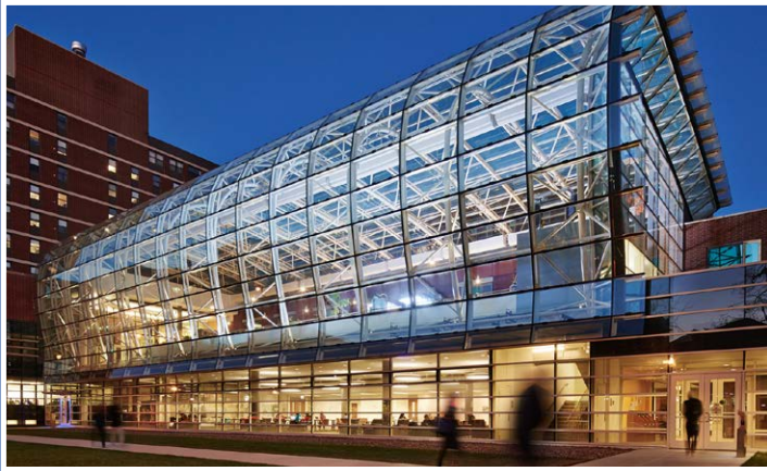
2014 SEA01 Best Project - Elliptically curved trusses rolled from 5" and 8" diameter AESS pipe for Institute of Environmental Sustainability at Loyola University. Chicago, IL
