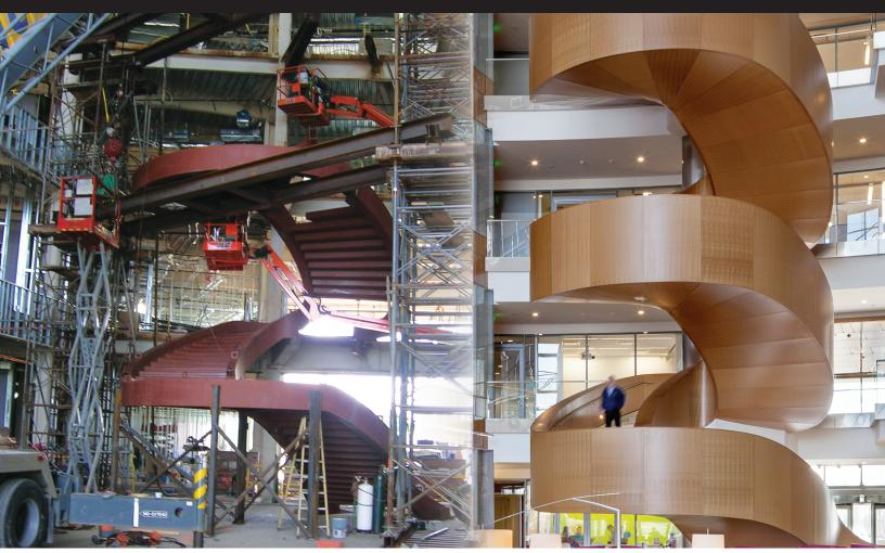
$5/8" \times 20" A572-50$  plate curved to make 20" x 8" welded box stringers. 15' radius (inside stringer) and 22' radius (outside stringer) for a multi-radial/flared orientation.
