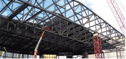
Each roof truss was erected on a shoring tower in two halves. Once a truss was completed and stabilized to the adjacent framing, the tower was moved to the next truss location.
