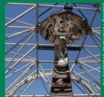
The erecting started with the omphalos or "belly button."
