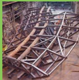
Littel Steel completely preassembled the structural steel.
