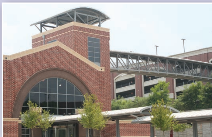
2006 IDEAS 2 Merit Award – 50 Tons of tube, angle and tee curved for the Multimodal Transportation Center. Athens, GA.
