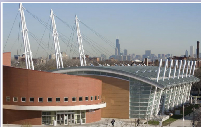
2004 EAE National Winner – 310 tons of beams bent including reverse curves for the Gerald R. Ford Center. Chicago, IL.
