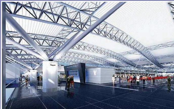
2002 EAE Merit Award – 400 tons of 16 inch pipe curved for JFK International Airport Terminal 4. Jamaica, NY.
