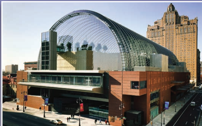
2003 IDEAS 2 National Winner – 300 tons of 5 inch square tubing curved 45° off-axis for the Kimmel Center. Philadelphia, PA.
