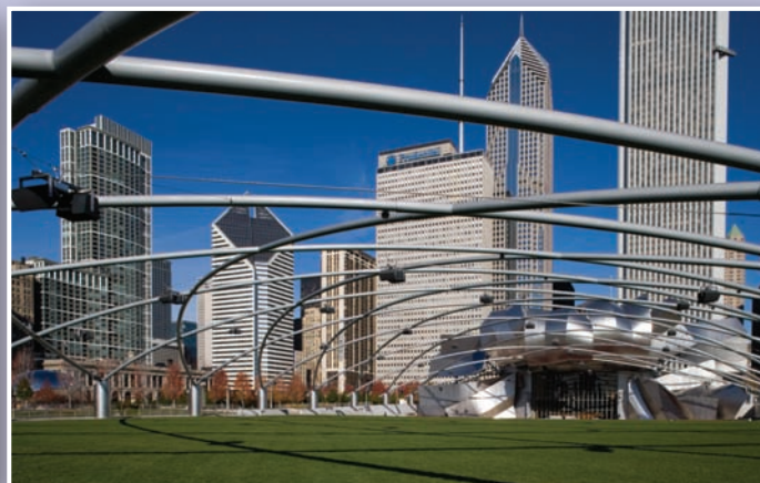
2005 EAE Merit Award – 570 tons of 12, 14, 16, 18, and 20 inch pipe curved for the Jay Pritzker Pavilion. Chicago, IL.
